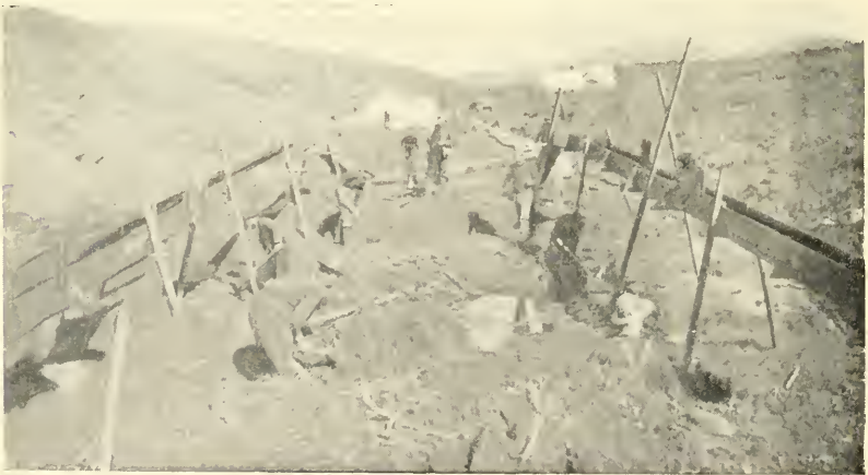
SLUICING ON CLAIM No. 5, ABOVE, ON ANVIL CREEK.
